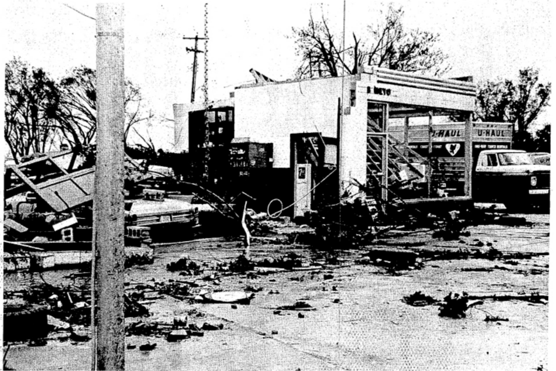
ONE OF OELWEIN'S business establishments leveled in the storm was Barney's Texaco at the north edge of the city. Fred's Super Valu, Sperry's Garage, and the Book & Art were also heavily damaged in the immediate area.
