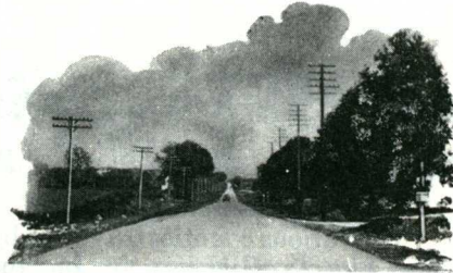
An example of the high grade concrete construction, 21 miles of which were completed last year in Indiana.
