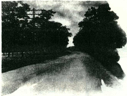
Where the Lincoln Highway is not brick or concrete in Indiana it is high grade macadam like the above. A type which necessitates excessive maintenance.
