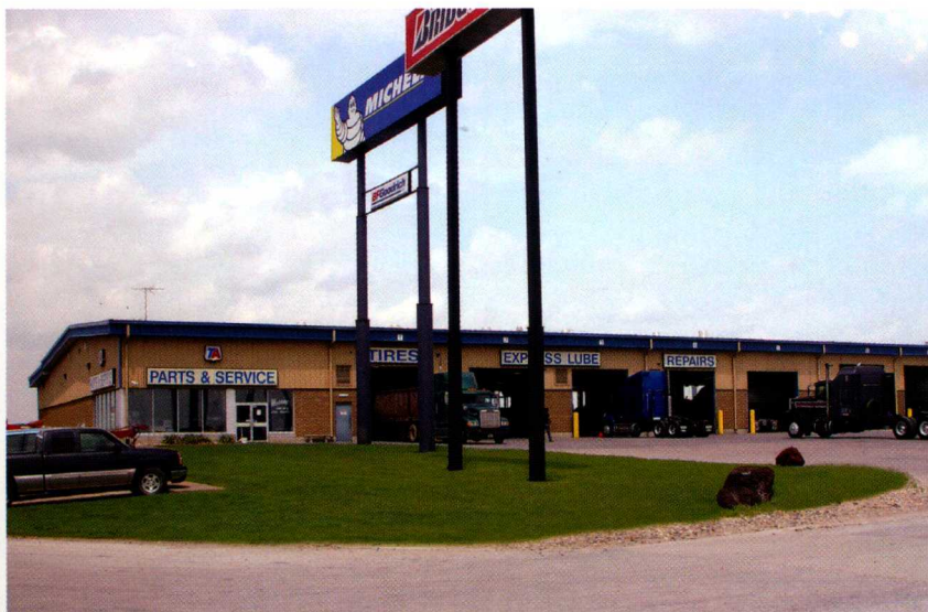
Iowa 80 Service Center with a whopping seven bays - 2004.
