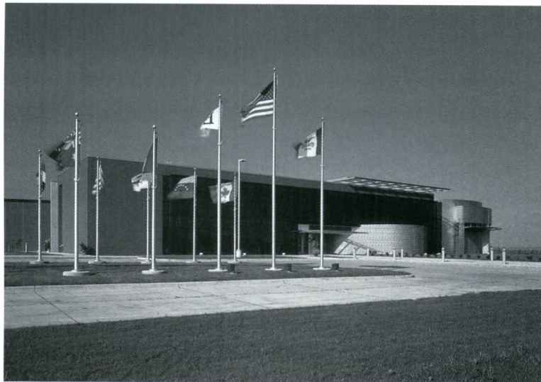
The 75,000-square-foot Global Pavilion includes a large arena, a training center with nine classrooms on two levels, and the Vermeer Museum.
