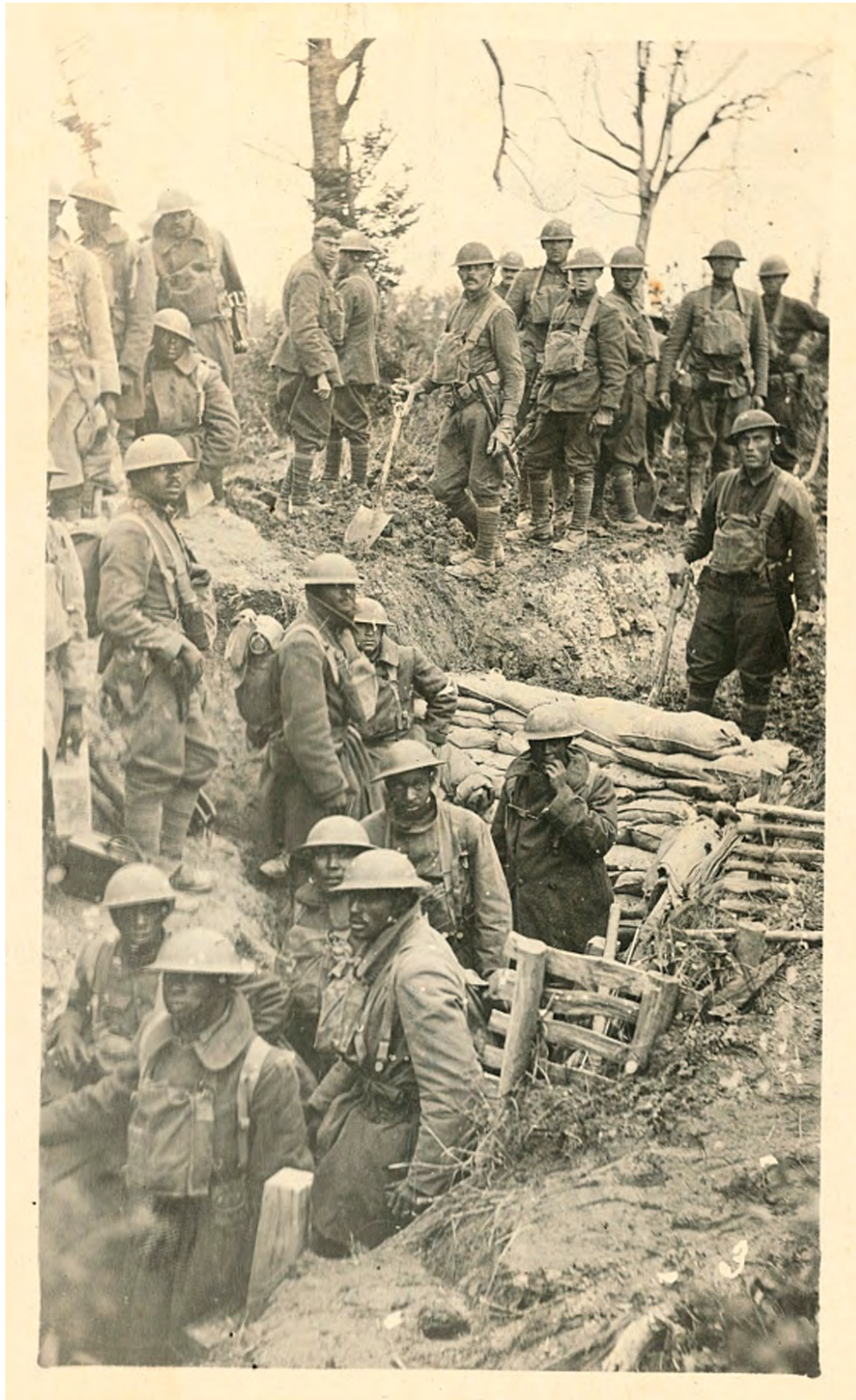
“302nd Eng. repairing road over trench and 92nd Div. (colored) machine gunners going into action, Argonne Forest, France,” 1918. Courtesy of Library of Congress
