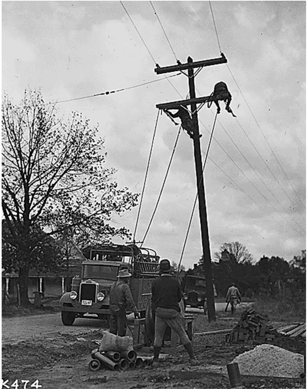
“REA; TVA; ‘Stringing rural TVA transmission line’,” 1933. Courtesy of National Archives
