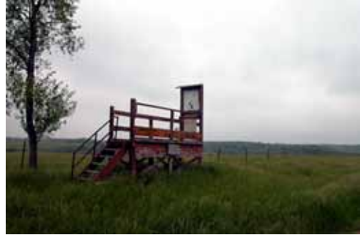
Seven-Mile Creek Viewing Platform.
