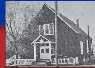
Adas Yeshurun, 1954. Adas Yeshurun operated from 1899 to 1955. It was one of about seven Orthodox synagogues in Sioux City through the early to mid-20th century. It closed in 1955 when the last five Orthodox synagogues merged into the United Orthodox Synagogue. Photo courtesy of Sioux City Public Museum
