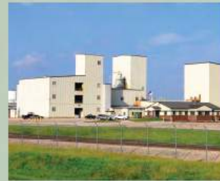
BIODIESEL PLANT NEWTON, JASPER COUNTY, 2019
