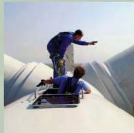
WIND TURBINE WORKERS ESTHERVILLE, EMMET COUNTY, ABOUT 2005
