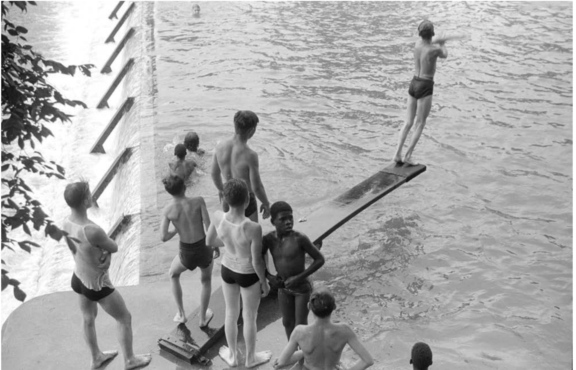
Courtesy of Library of Congress, Roskam, Edwin, "Swimming pool created by CCC (Civilian Conservation Corps) dam, Huntingdon, Pennsylvania," July 1941
